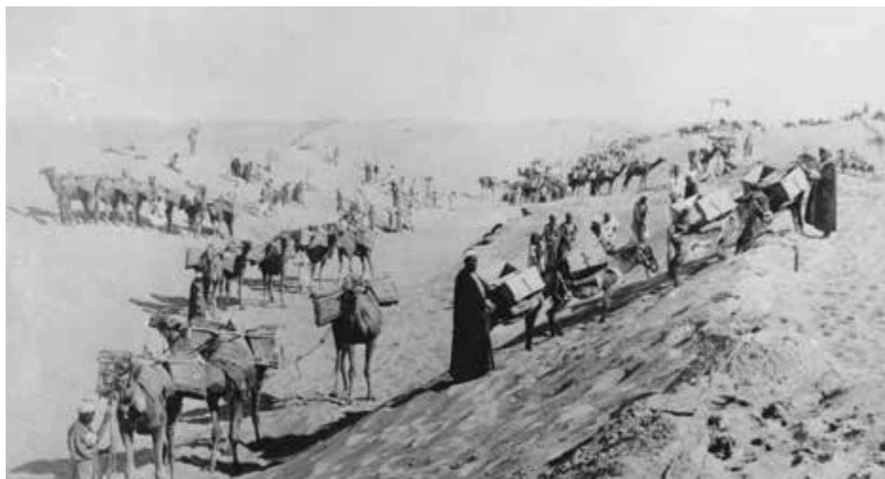
Hundreds of thousands of workers were involved in digging the canal, equipped only with picks and shovels, before machines arrived at the site © D.R.
