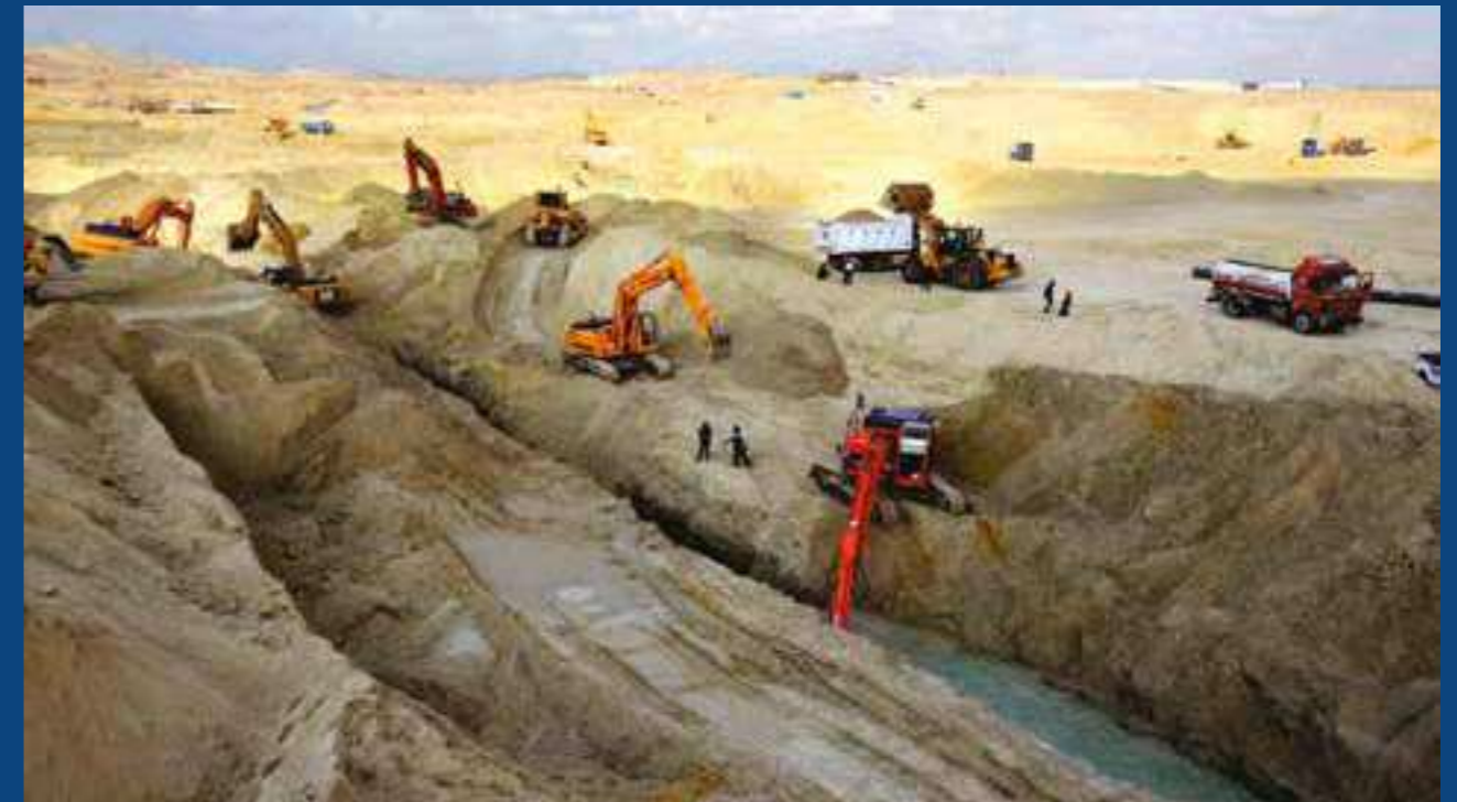
Most recent works on the Canal, during the extension.
