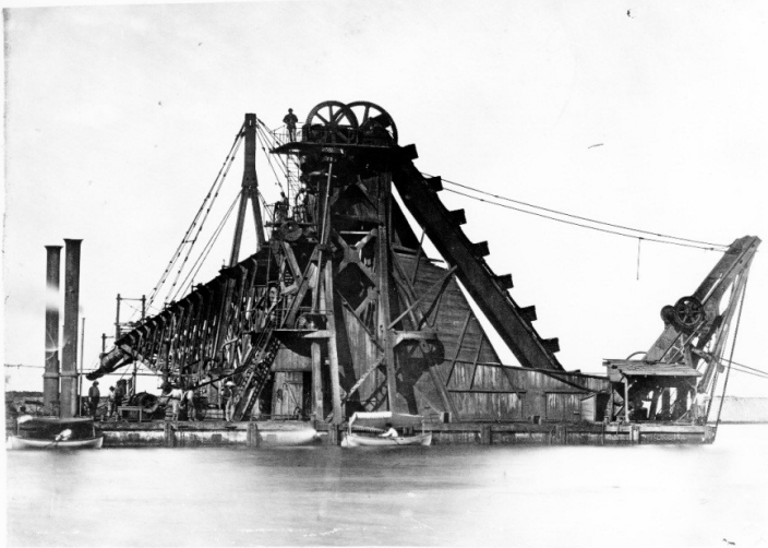
Dredge used on the Suez Canal in the 1870s. H. Arnoux, 1869 © Souvenir of Ferdinand de Lesseps and the Suez Canal
