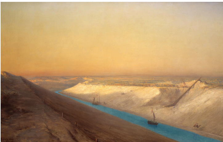
"The Worksite" by François Pierre Bernard Barry © Souvenir of Ferdinand de Lesseps and the Suez Canal / Lebas Photographie Paris
